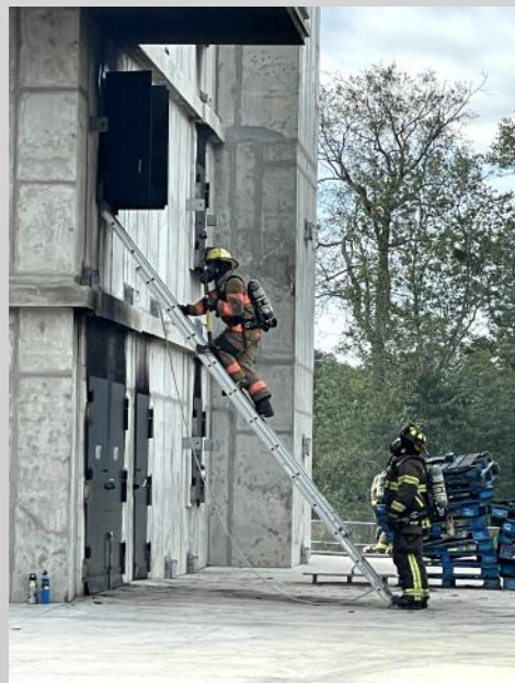
RFTC Burn Building
